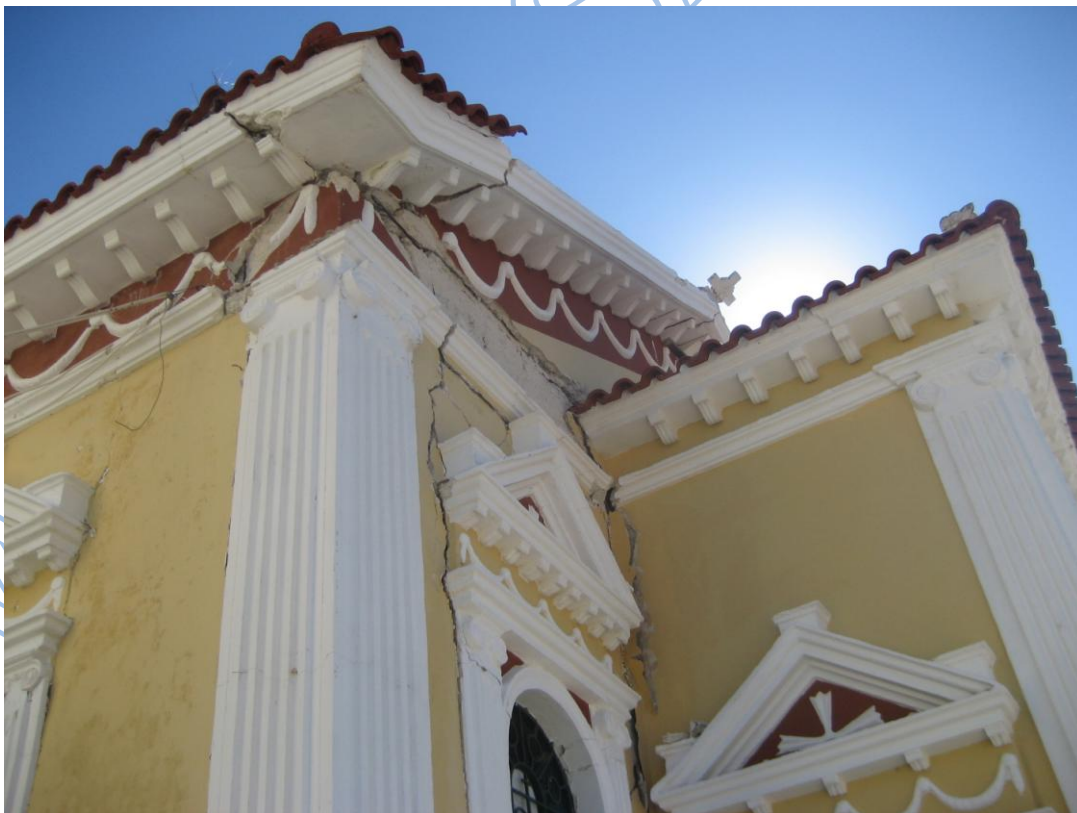
Photos 3.57, 3.58. Temple at the southern villages of Paliki peninsula as damaged during 26-1-2014 (up) and during 3-2-2014 (low) earthquakes.
