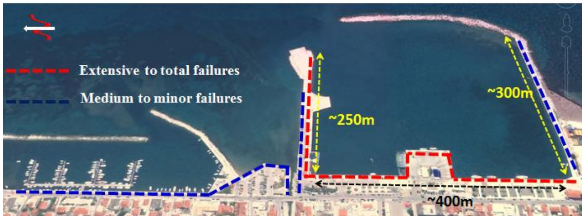
Figure 2.14. General outline of the severity of damage induced by the second earthquake of 03/02/2014 at the main piers of Lixouri port.
