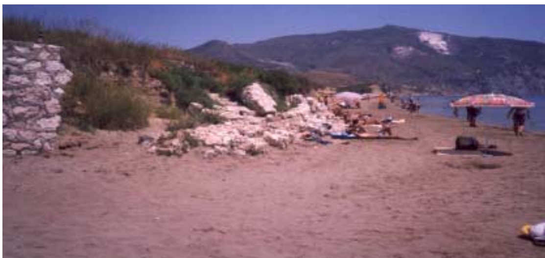
Illegal walls collapsing on to the narrow beach of Kalamaki.
