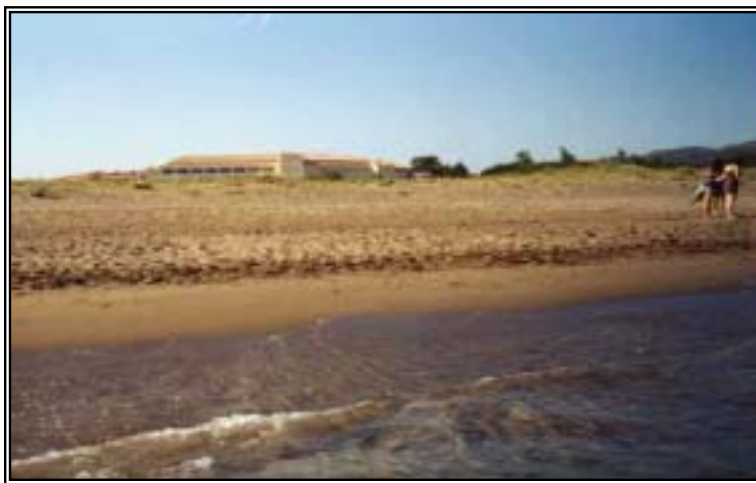
Photo No. 3: New two storey hotel overlooking Kalamaki beach (16/06/01).
